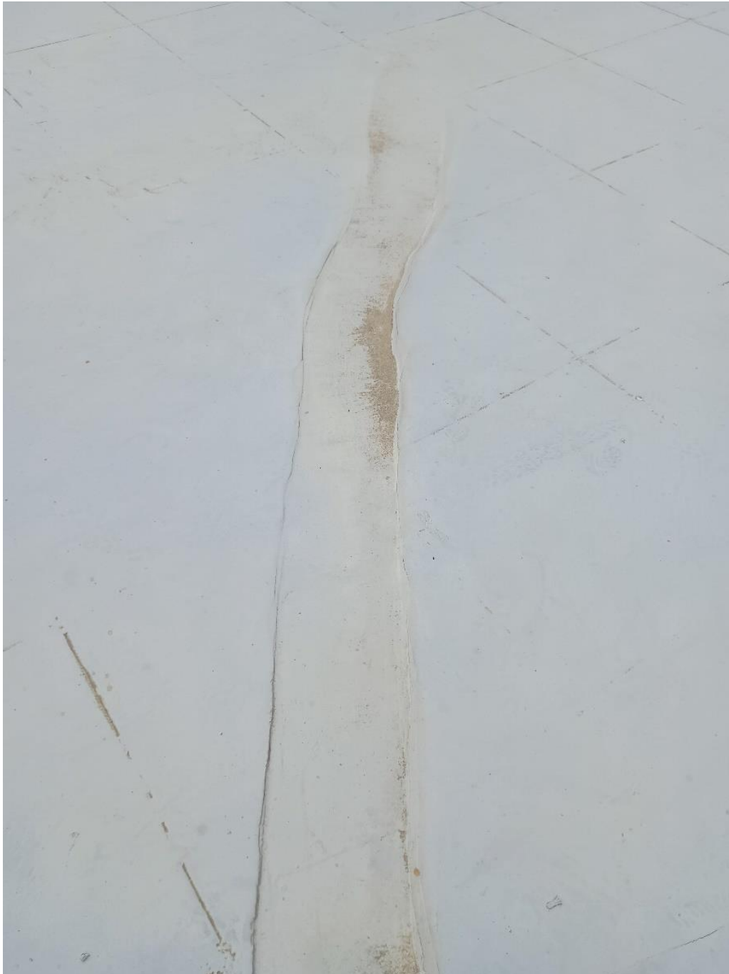
Figure 13: : Roof coating breakage
